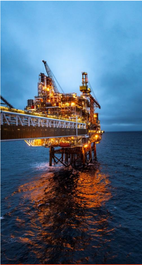
Talbot: 1 st of 3 development wells successfully completed
