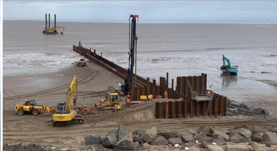
Cofferdam complete on the beach at Easington – June
