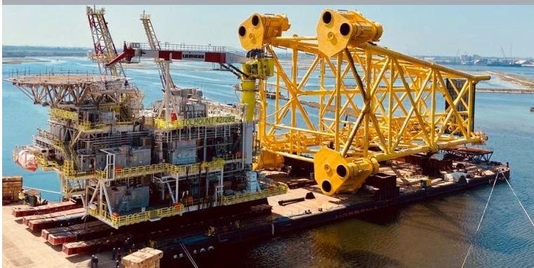
Pile offloading on to transport barge
