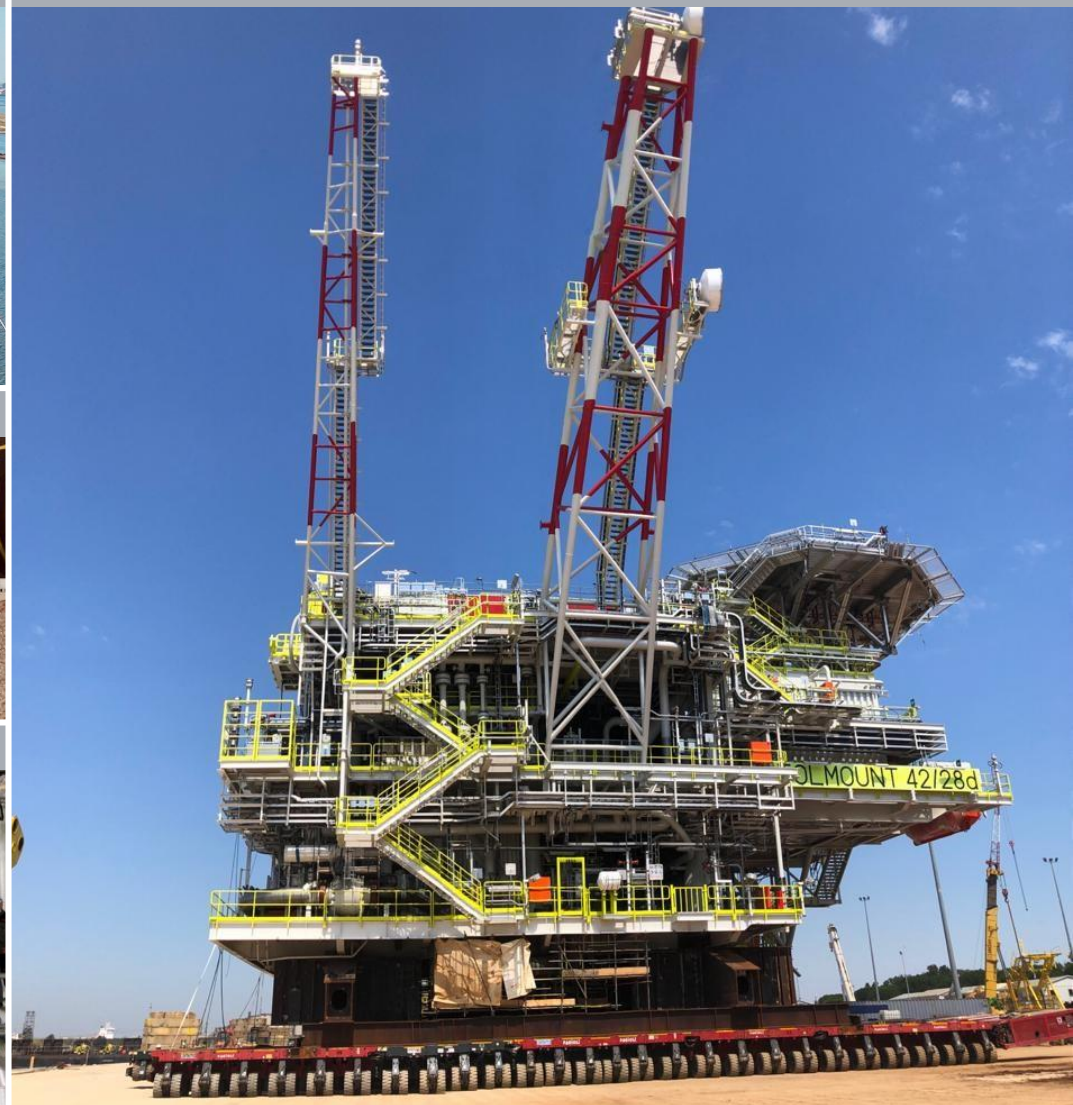
Topsides transportation to barge
