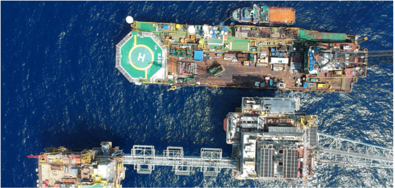
Anoa - Anoa Gas Exploration (AGX) Complex, offshore Indonesia
